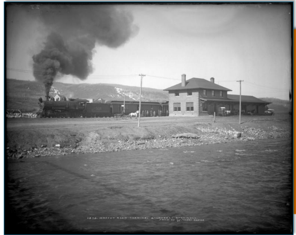
Photograph 8. Exterior view of "Moffat Road" Denver & Salt Lake Railroad station, Steamboat Springs, Colorado; engine and passenger train parked at depot, "The Royal" horse-drawn wagon & others; Yampa River, foreground (1913-1915) (Louis Charles McClure, Denver Public Library Special Collections, MCC-1272).
