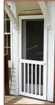
Photograph 22. Example of a residence with an updated screen door. 16
