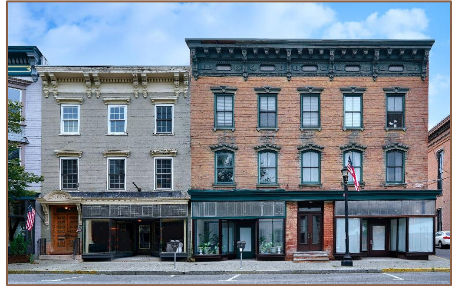
Photograph 28. Example of a row of commercial buildings that have maintained their significant architectural features. 20
