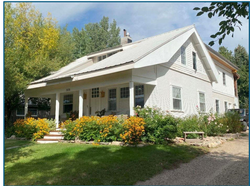
Photograph 58. Local example of a Mass-Planned style residence with a rear addition.
