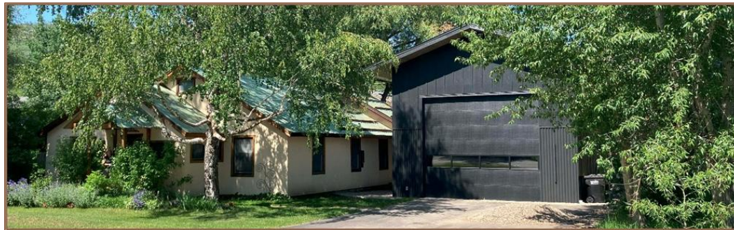
Photograph 39. Example of a non-historic, detached garage next to a residence with incompatible design, scale, and sitting.
