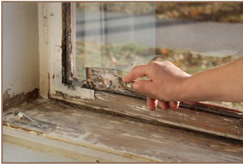
Figure 3. Window restoration. Deteriorated paint does not always indicate a window is beyond repair. 6
