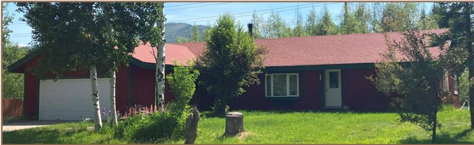
Photograph 21. Ranch style residence with original door placement and sizing.
