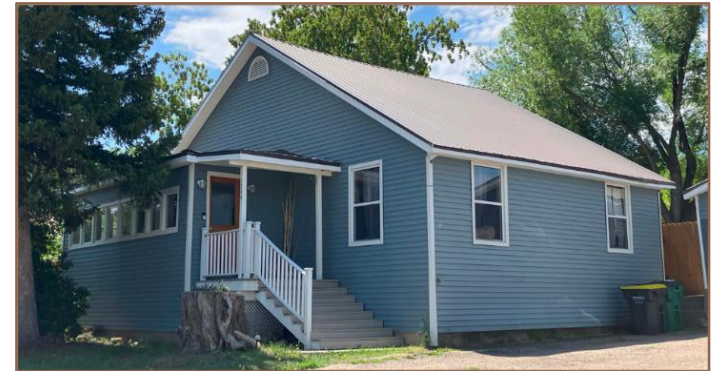
Photograph 34. Example of an enclosed front porch.
