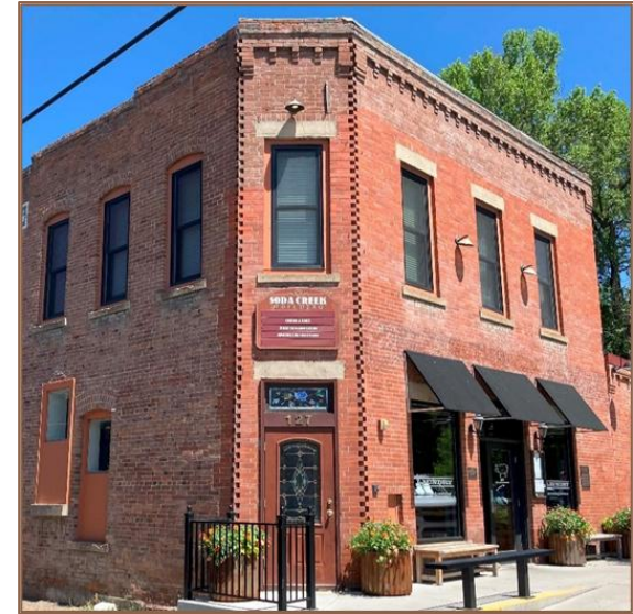
Photograph 26. An example of a building with brick sheathing that has been partially replaced. It maintains the historic running bond pattern and brick size and materials, while not obscuring that it is newer brick through its coloring.
