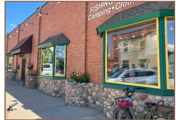
Photograph 27. Non-original river rock planters along the side of a historic brick building.
