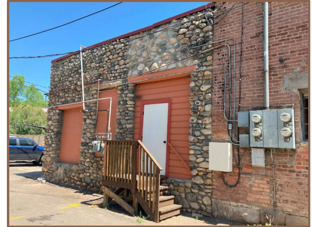
Photograph 29. Example of an addition with river rock façade facing attached to a historic brick building.
