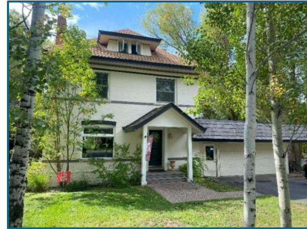
Photograph 68. Local example of an American Foursquare form.
