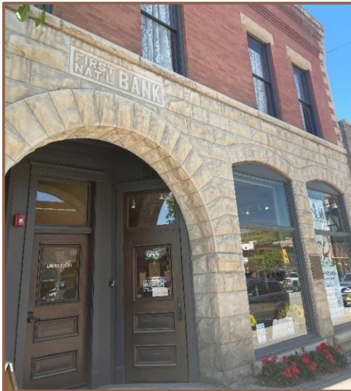
Photograph 3. The First National Bank Building.
