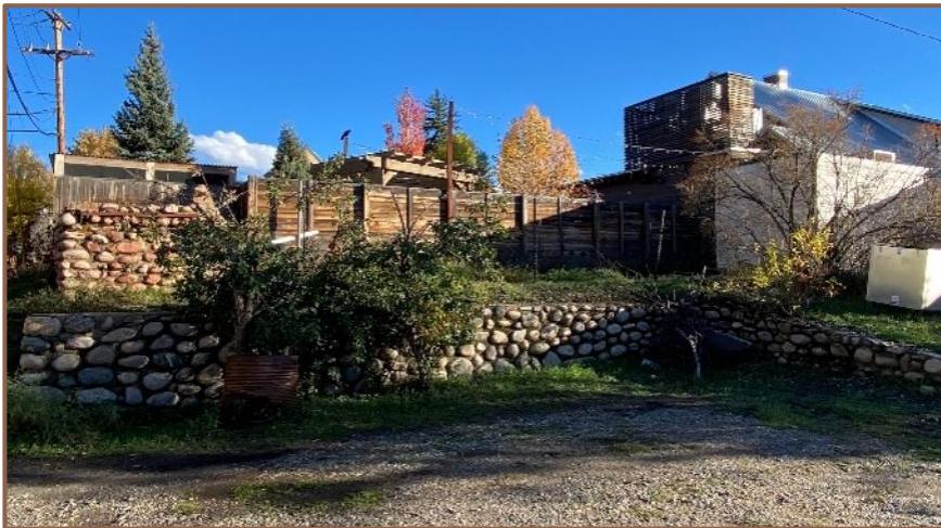
Photograph 31. View of river rock features in an alley.
