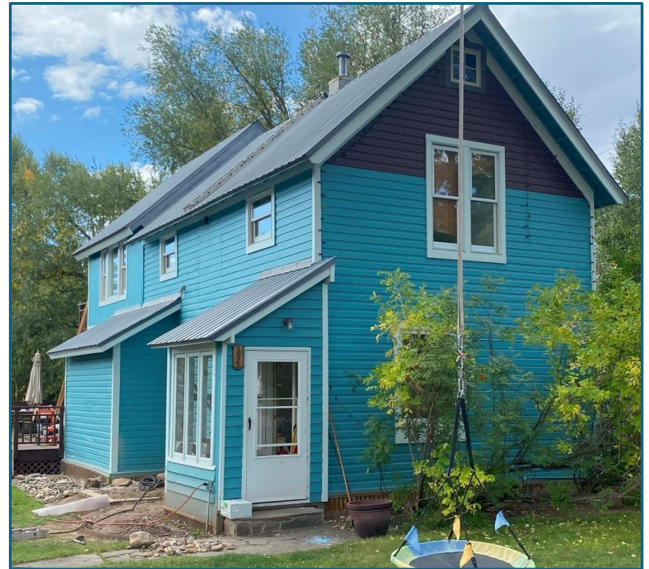
Photograph 57. Local example of an I-House style residence with an enclosed porch and an addition.
