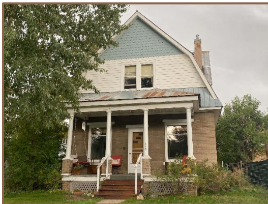
Photograph 10. Dutch Colonial Revival style building with preserved windows
