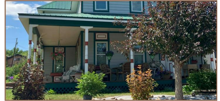
Photograph 33. Preserved wrap around porch with original turned decorative posts.
