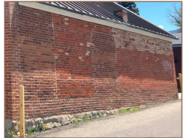
Photograph 30. Example of a historic building with replacement brick and roofing around historic elements.
