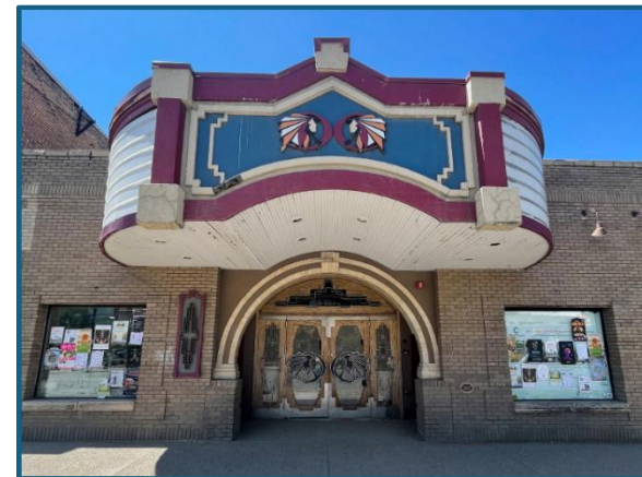
Photograph 69. Local example of an Art Deco style commercial building.
