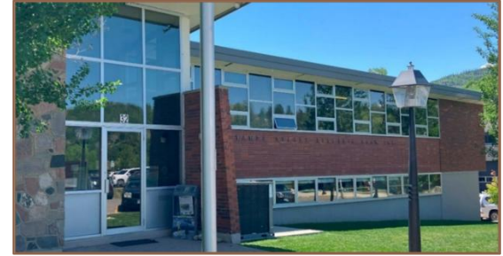
Photograph 12. Historic mid-century building with preserved historic windows.
