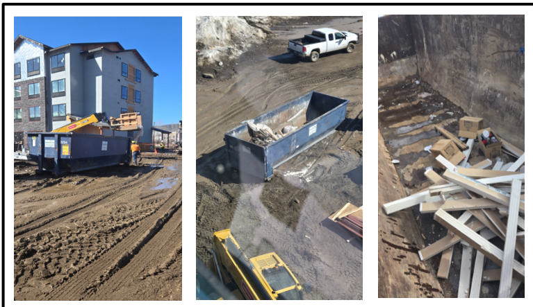
Image 12: Site Trash Dumpster with cardboard, soft plastics, and cutoffs of drywall. (March 2025)
