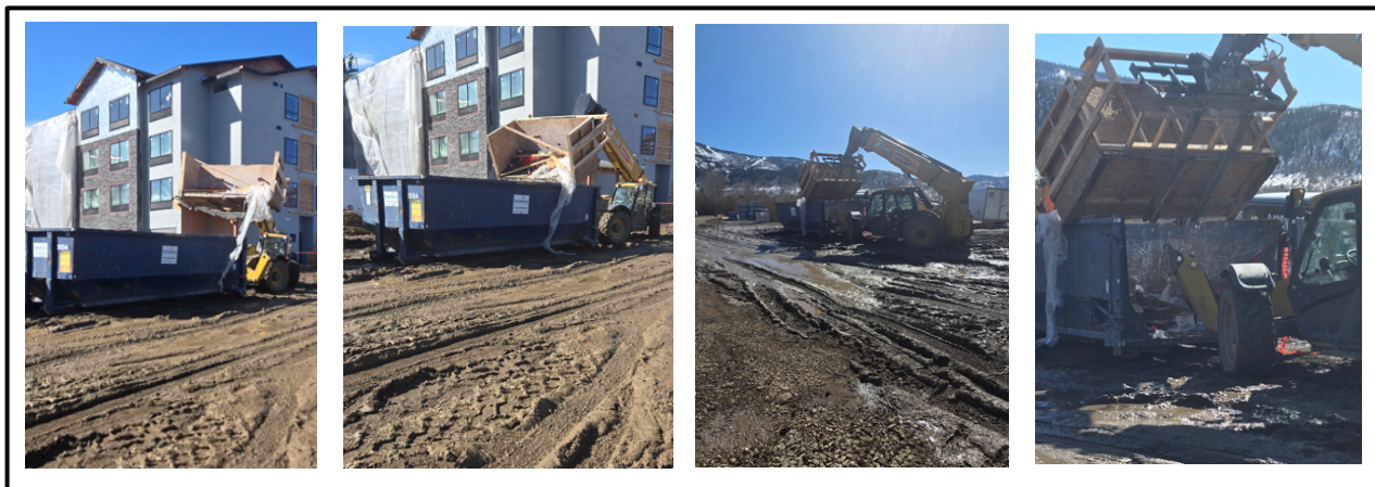
Image 13: Site Trash Dumpster and Trash Box (March 2025)
