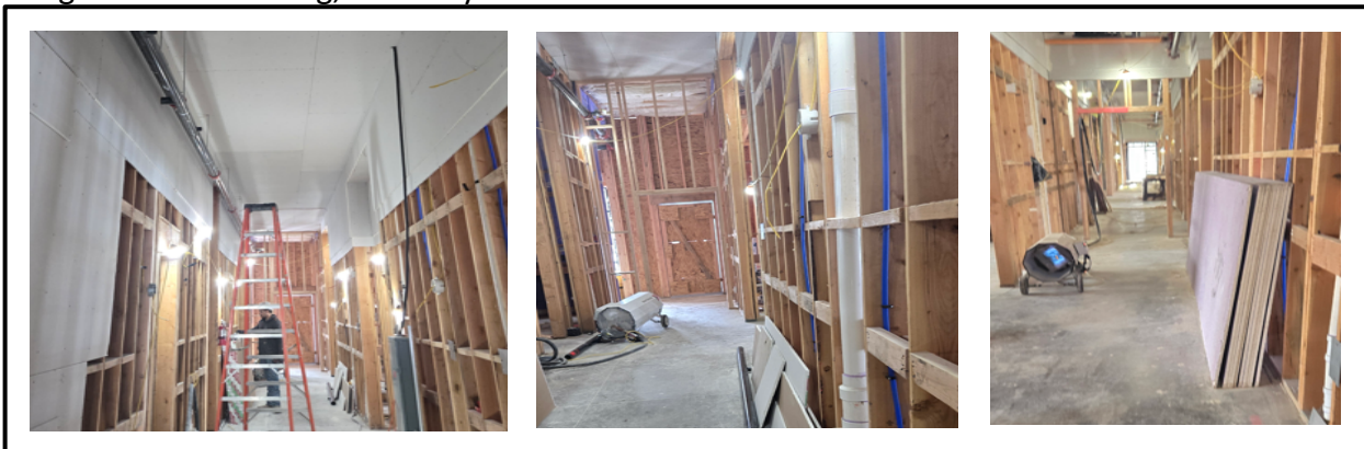
Image 1: Floor Framing, February 2025
