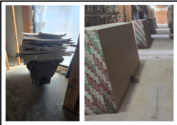
Image 5: Gypsum cutoffs and boards
