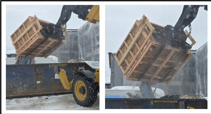
Image 7: Gypsum Material and Disposal (February 2025)
