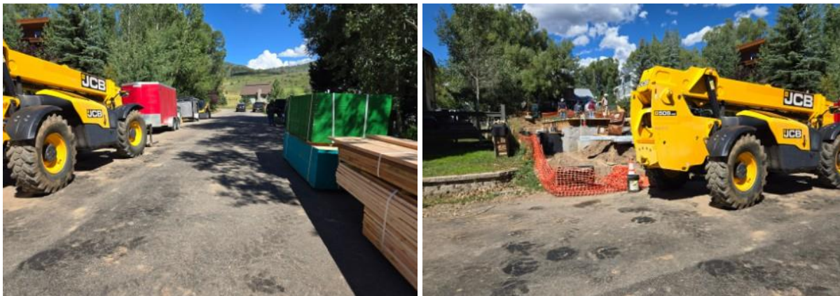
Image 24: Fox Construction August Site Space, street view of construction site.
