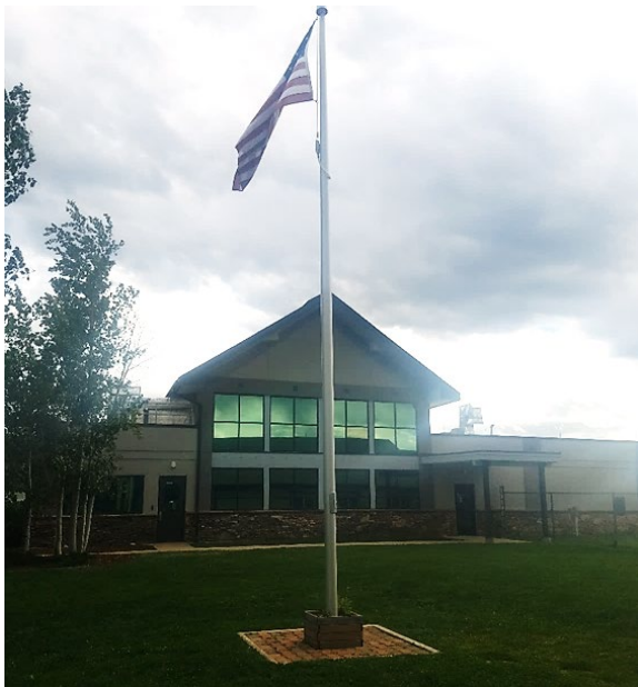
Figure 1.11: Airport Office Building (AOB)
