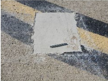
Small Patching (Sample Unit No. 01)
