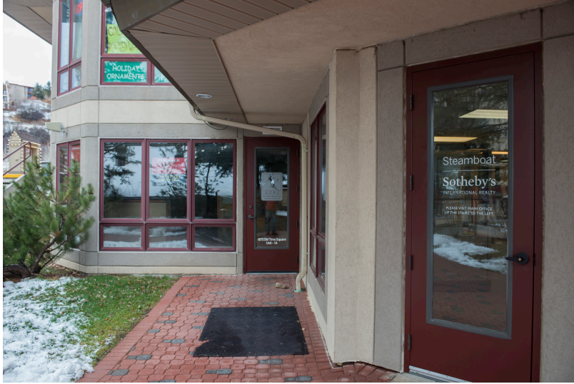
Entrance View (from path to pool). Adjacent office entrance.
