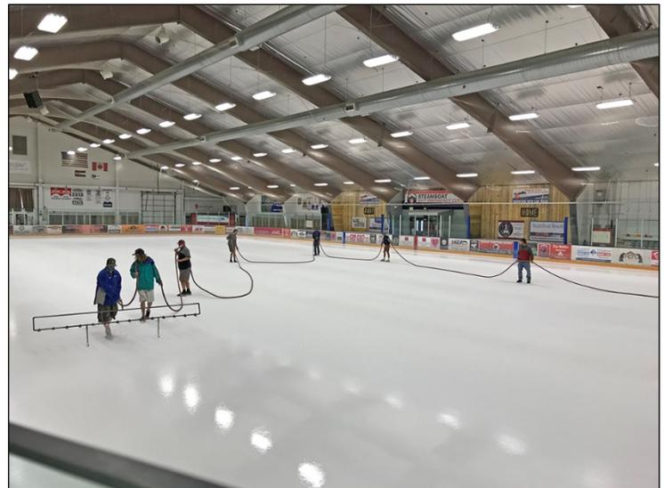
The process to set the ice and paint the lines takes between seven to ten days to complete and is currently underway. Approximately 20,000 gallons of water are used to build the 1.5 inches of ice on an Olympic-size sheet, enough to fill 150,000 16oz glasses. Water is put down in layers and allowed to freeze before the next layer is applied. Mid-way through the laying process, lines are painted before additional water is applied.
